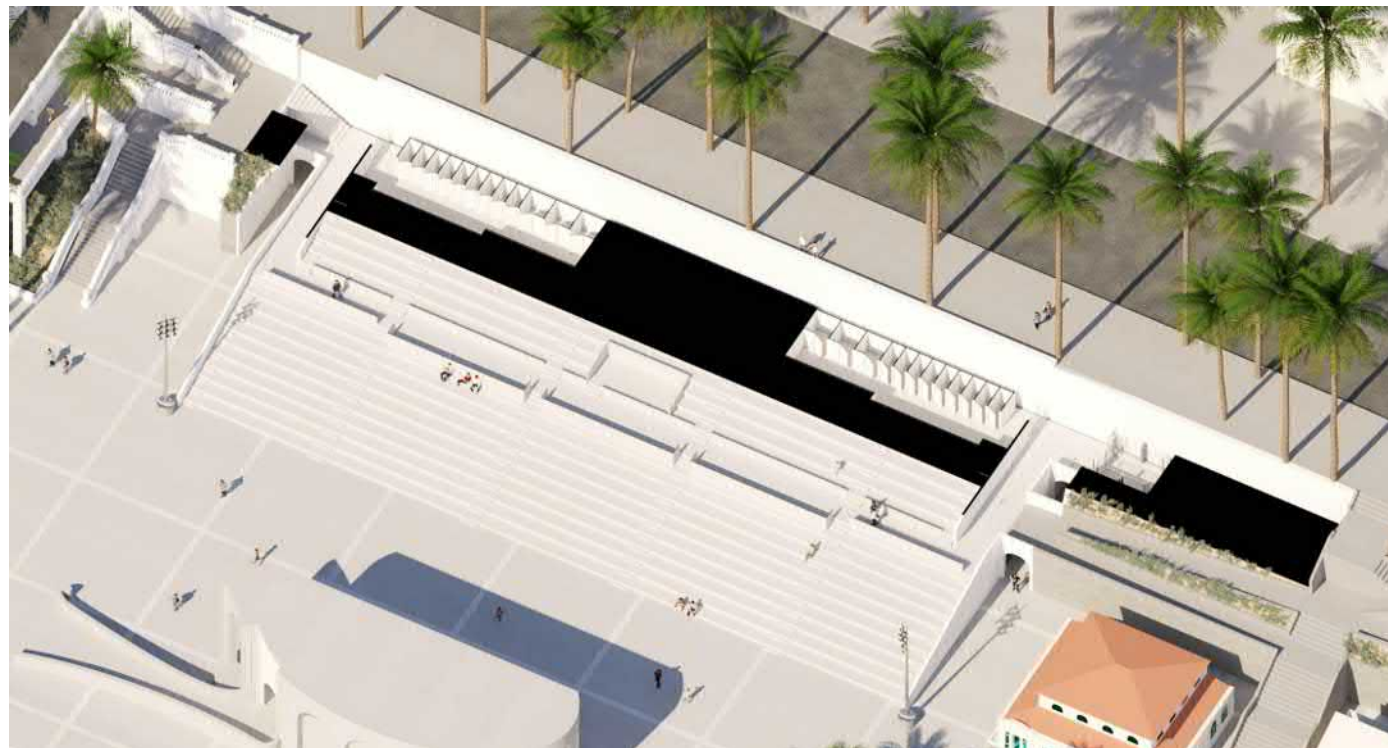
MID LEVEL A cross aisle at the Mid Level connects the Pier Bridge Stairs and south site ramp entrance/exits. Additional wheelchair seating and the Sound Mix station are also located at the Mid Level. Restrooms, at this level, serve both sides of the amphitheater and are built below the amphitheater seating. A two-stop amphitheater elevator connects the Strand level and Mid Level of the structure.
