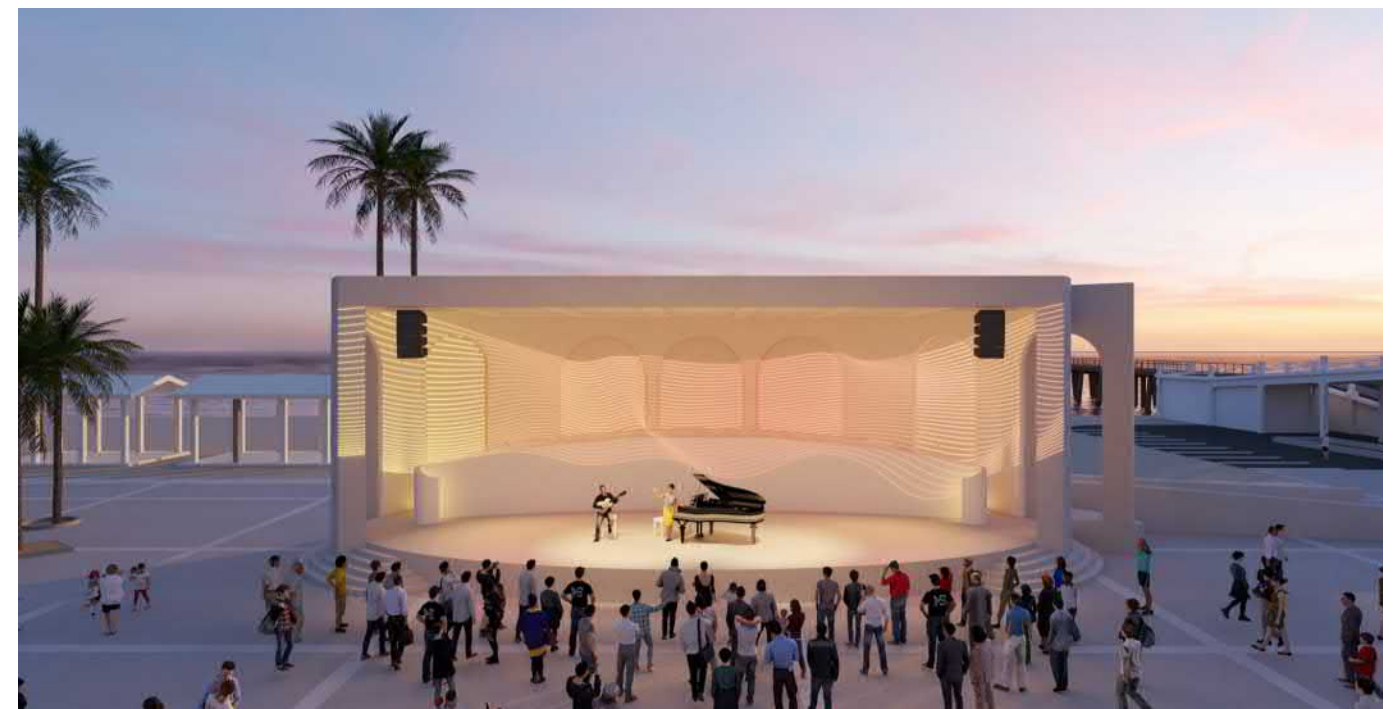
PROPOSED BANDSHELL The stage area is fully covered and the roof structure includes built-in infrastructure to support lighting and audiovisual systems. With this structure, there is no need to construct stage rigging for community events and performances.
