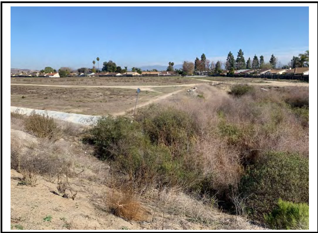
Photo Point 10. Photo taken January 8, 2021 facing east showing vicinity of Pala Road ditch including the outfall of brow ditch along toe of SLR berm that drains into adjacent riparian area.
