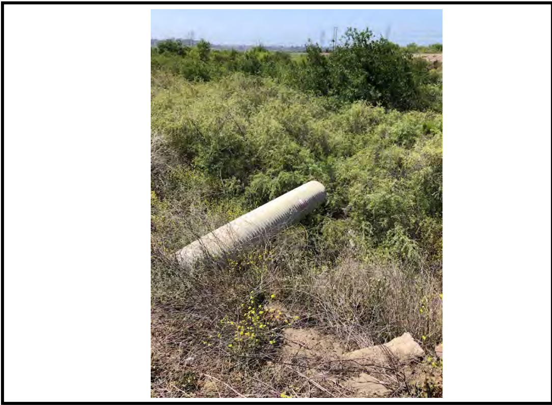
Photo Point 9. Photo taken January 8, 2021 facing south showing Pala Road ditch outfall.
