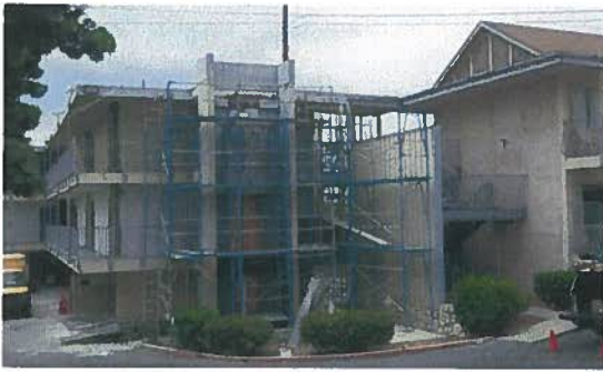
Existing Motel – East Elevation
