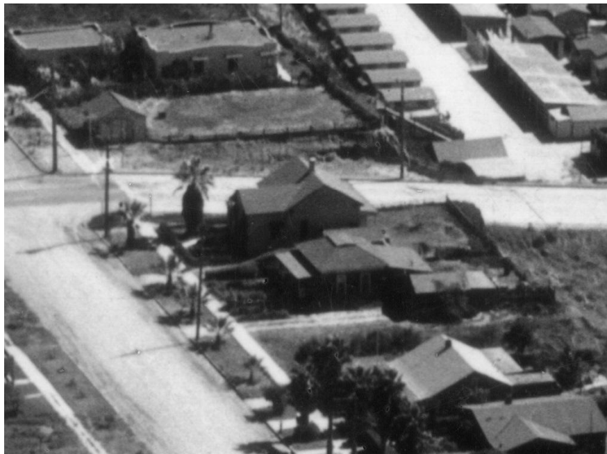
Closer view of 601 North Pacific Street, devoid of "circle window" on north facing facade
