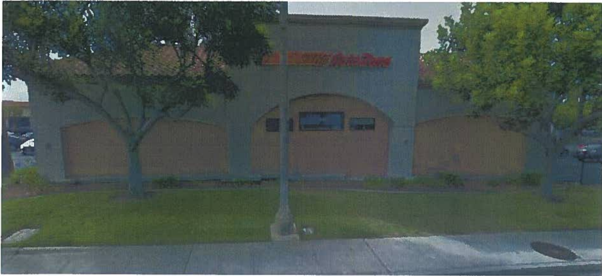
Existing South Elevation facing Mission Street
