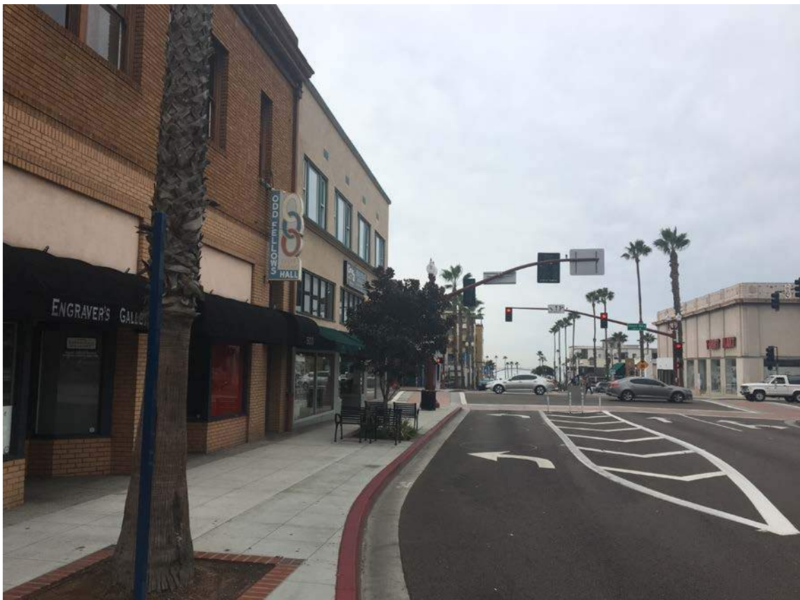
Photo 4: View of Mission Avenue with future CVS Pharmacy building to the left, facing Southwest
