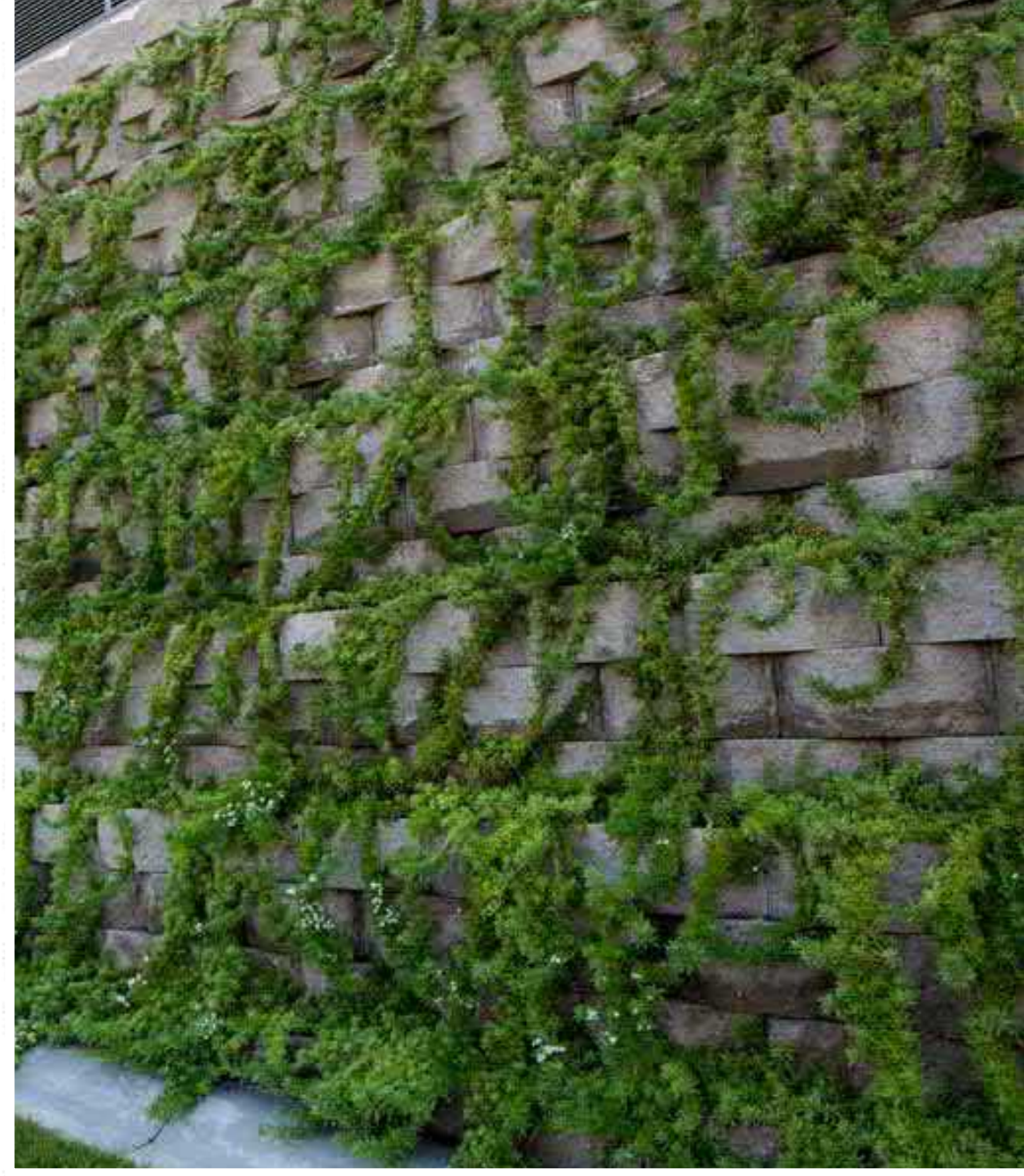
Sample of a planted retaining wall
