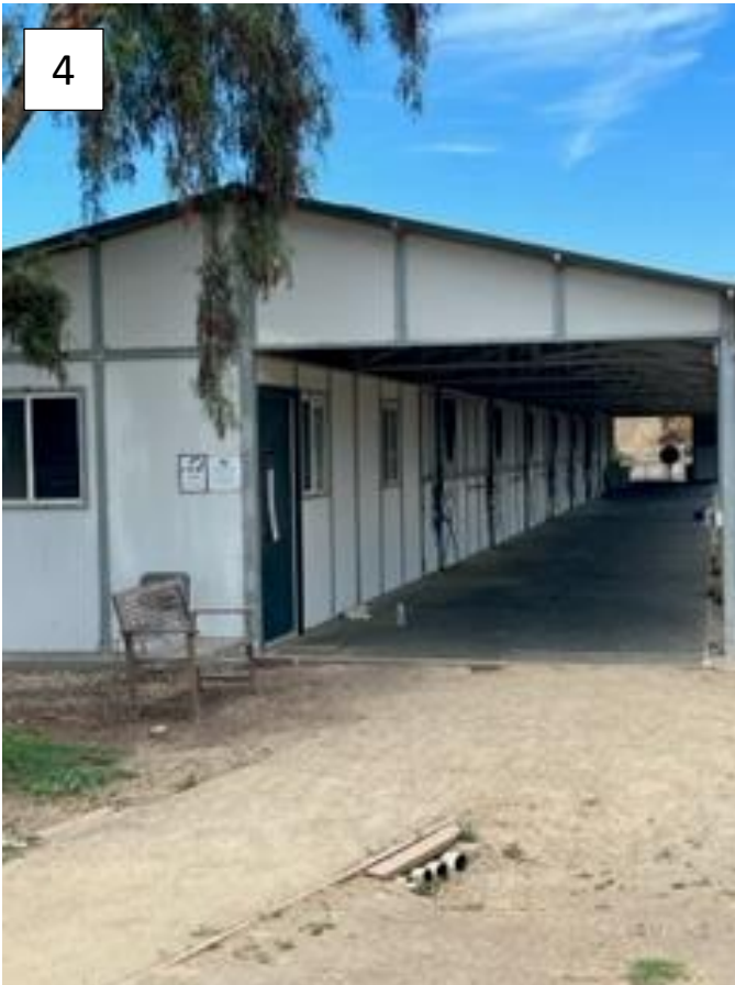
Stalls at existing facility
