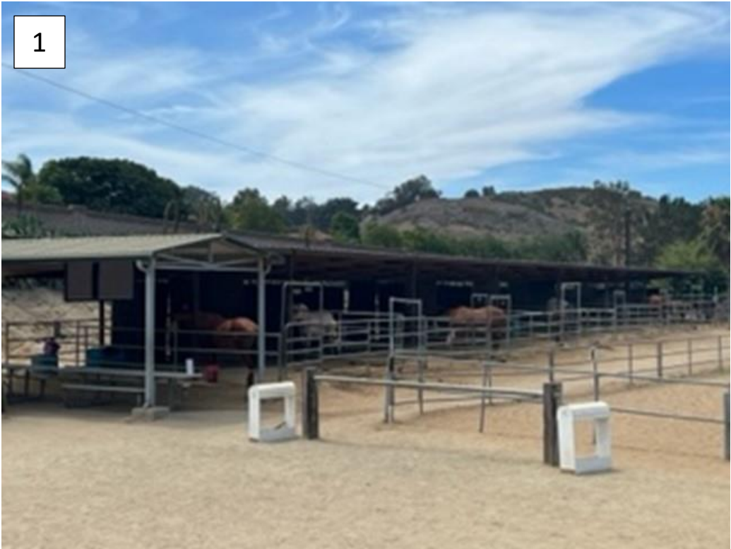
Stalls at existing facility
