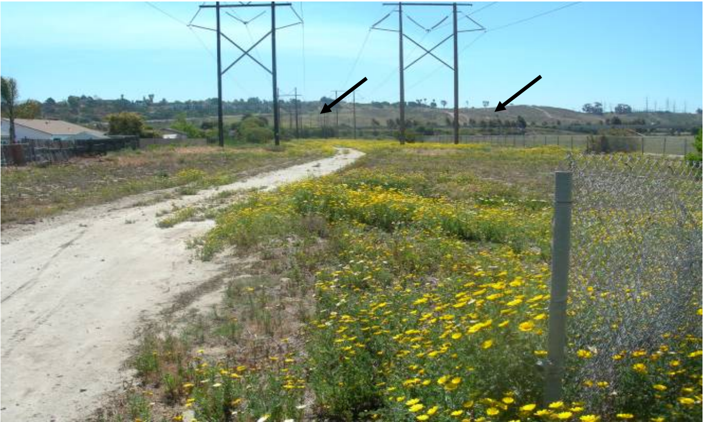
SDG&E Transmission Line along the eastern boundary of Pavilions project site looking south. Occupied gnatcatcher habitat is in the background (arrows) on the south side of SR 76.
