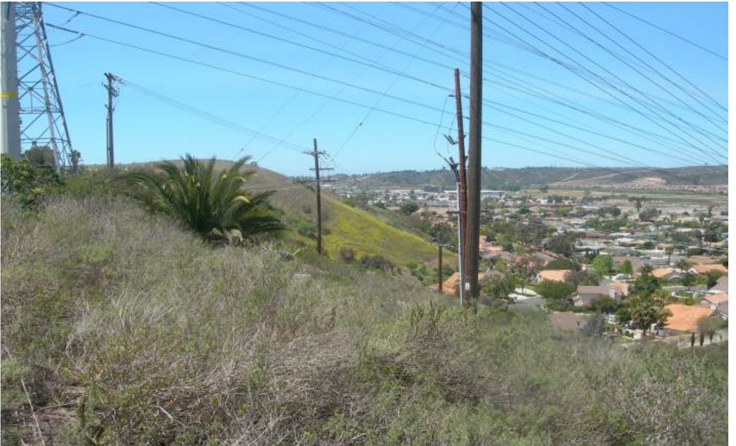
Western habitat linkage looking west from major transmission line corridor near substation.
