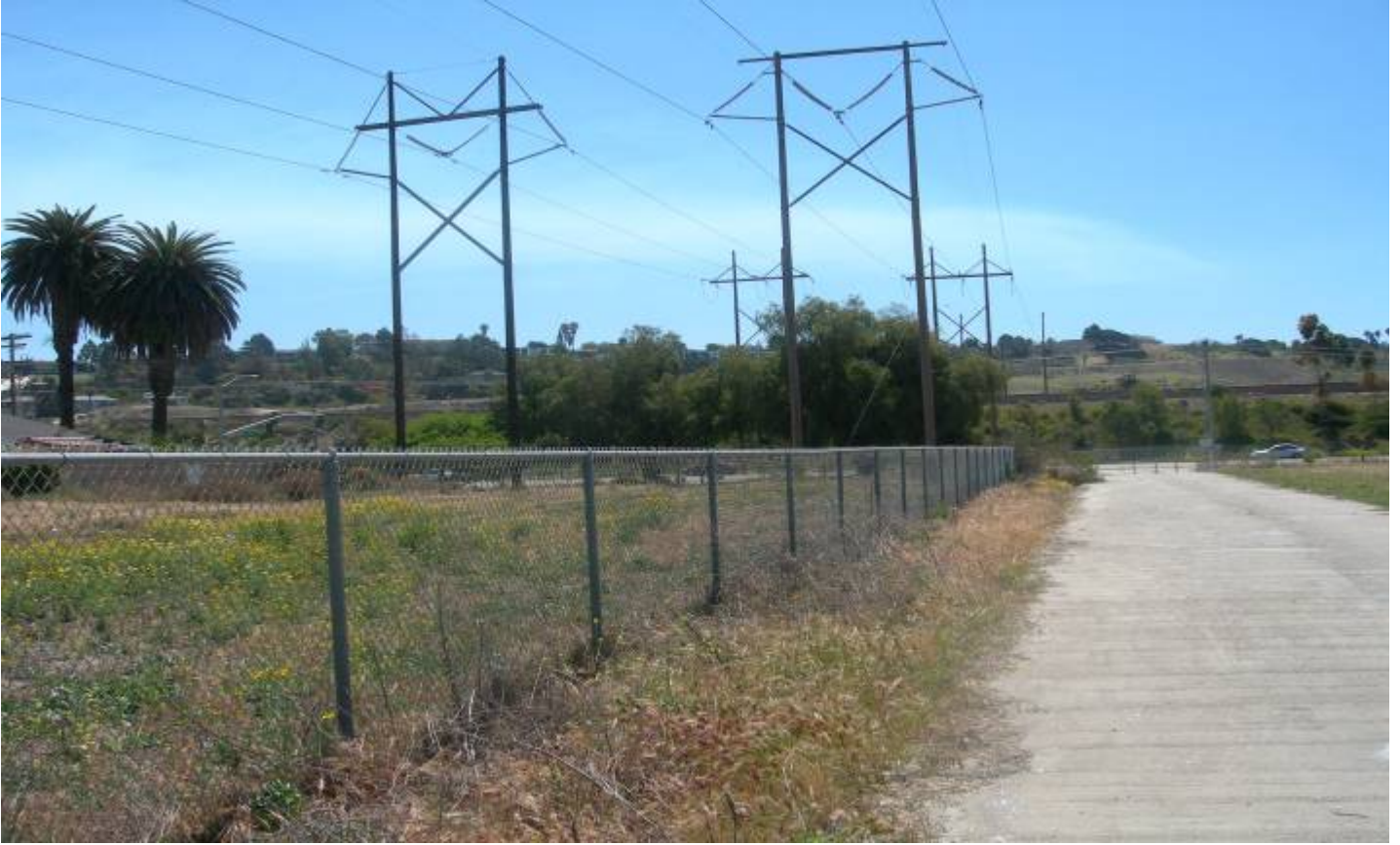
SDG&E Transmission Line along the eastern boundary of Pavilions project site looking south. Note concrete-covered storm drain.
