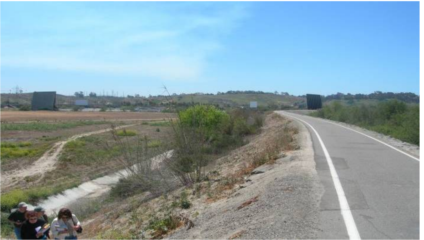
Looking west along river levy at north end of Pavilions site.
