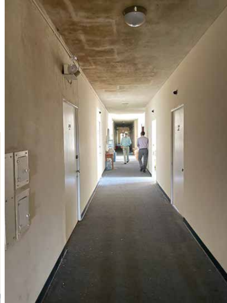
Main Hallway - 2nd Floor
