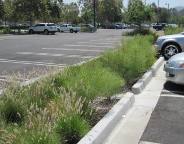
Figure 2. Bioretention in the parking lot of the LA Zoo.
