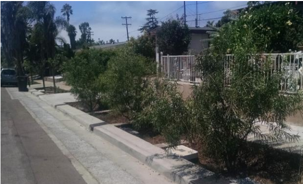
Figure 1. Bioretention incorporated in a green street in San Diego, CA.
