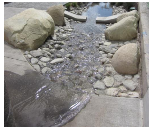
Figure 7. Example of a forebay as pretreatment for a bioretention area.
