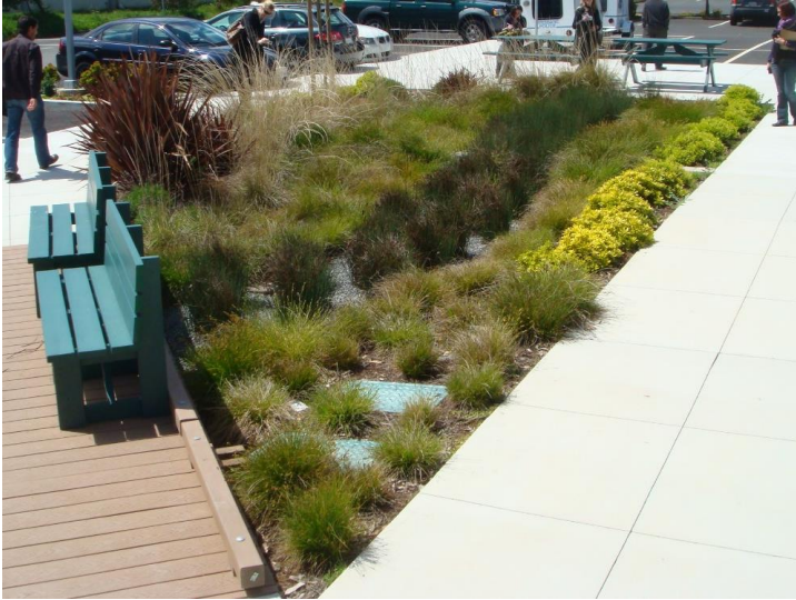
Figure 4 Bioretention in San Francisco, CA. Source: Jim Hook
