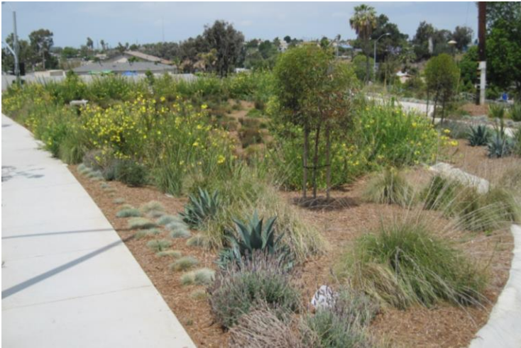
Figure 3. Bioretention in a landscaped area in San Diego, CA.
