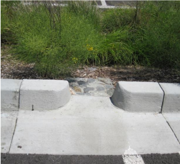
Figure 5. Example of an open curb cut.
