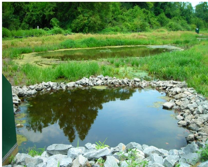
Figure 3. Example of a forebay as pretreatment for a constructed wetland.
