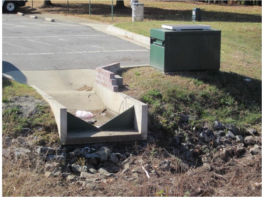
Figure 4. Example inlet structure.
