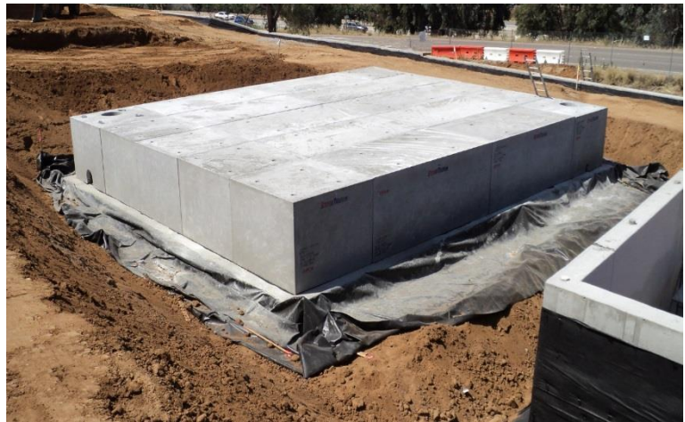
Figure 3. Subsurface design of an extended detention basin, during construction.
