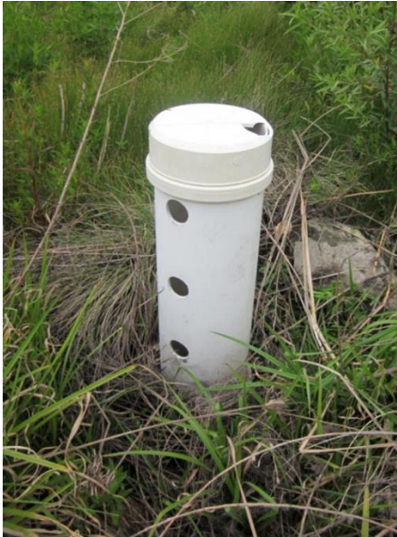
Figure 2. Variable flow outlet structure.
