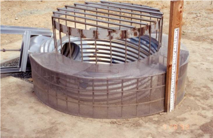
Figure 1. Example of outlet structure.
