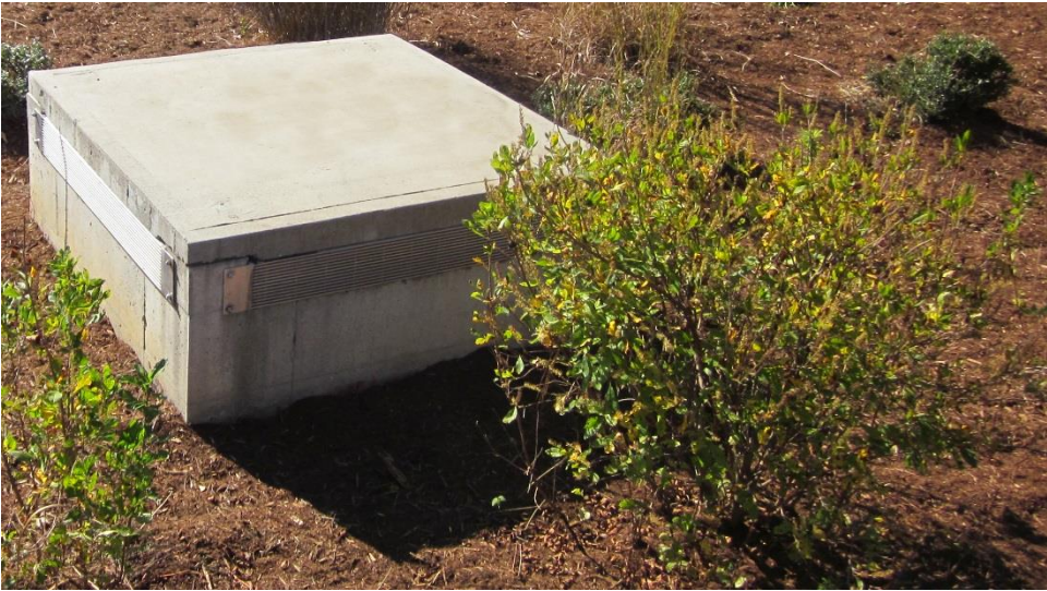
Figure 5. Outlet structure with a 5mm screen.
