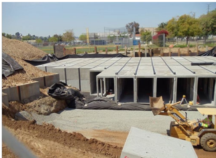
Figure 1. Subsurface design of an infiltration basin, mid-construction.
