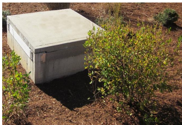
Figure 5. Example of an outlet with 5 mm screen.
