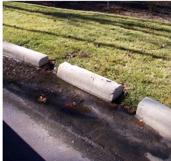
Figure 4. Example of filter strip as pretreatment
