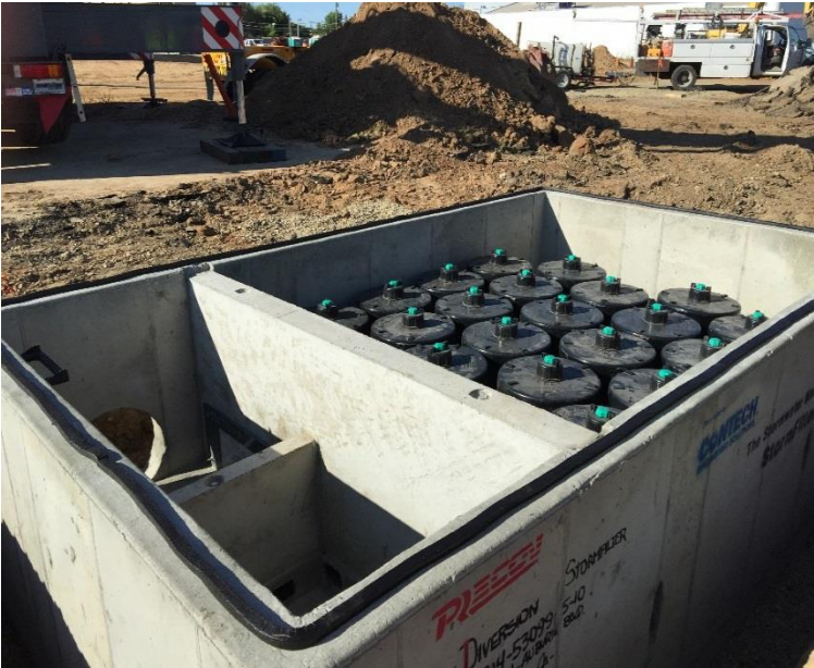
Figure 1. Stormwater media filter vault, mid-construction.
