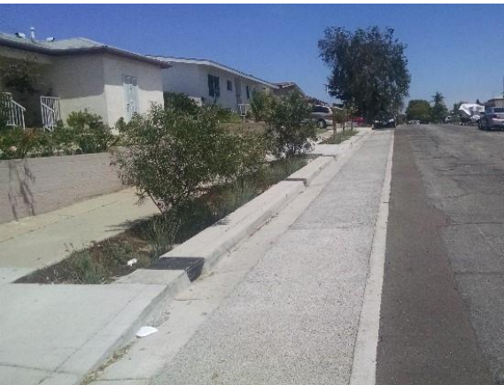
Figure 1. Pervious concrete parking lane in San Diego
