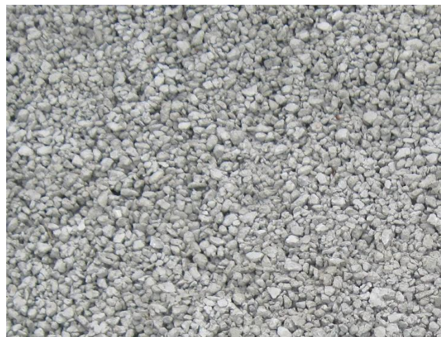
Figure 4. Example of pervious concrete.
