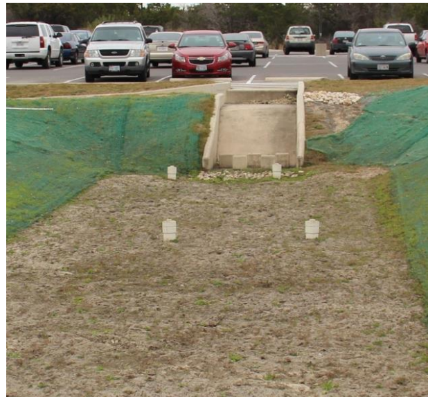
Figure 2. Example surface sand filter inlet.
