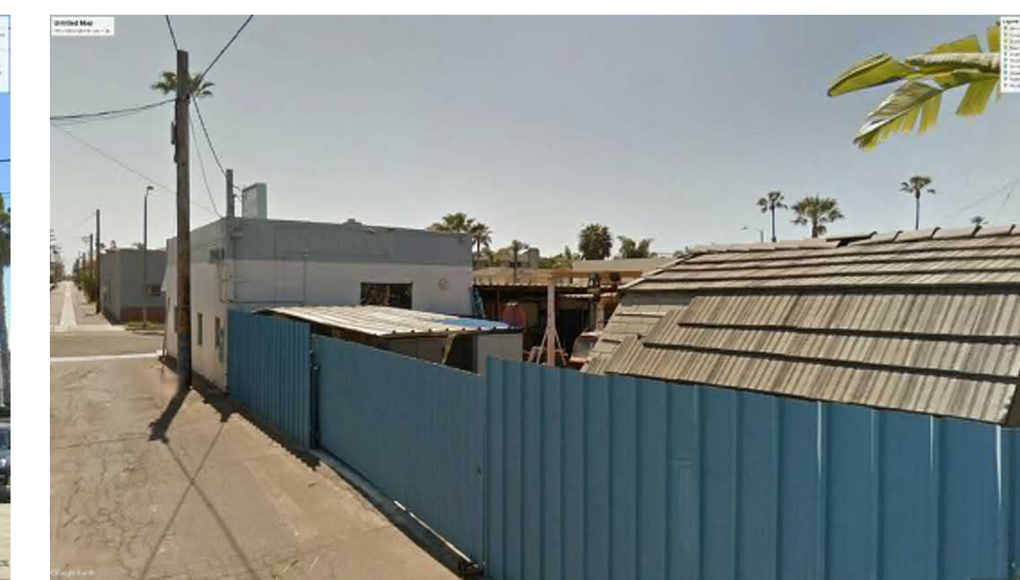
5. ALLEY LOOKING SOUTH
