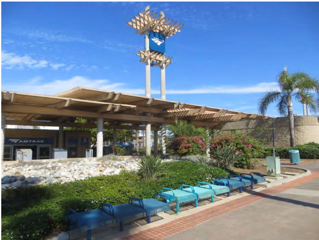
Photograph 8: Facing north at the location of the proposed future 4-story NCTD headquarters building, which will replace the existing office building (Photograph 1) as well as the administration building located on Mission Avenue.
