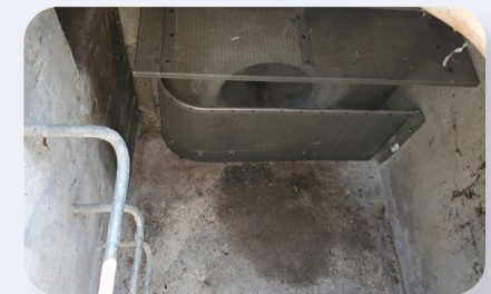
After FCD Installation
