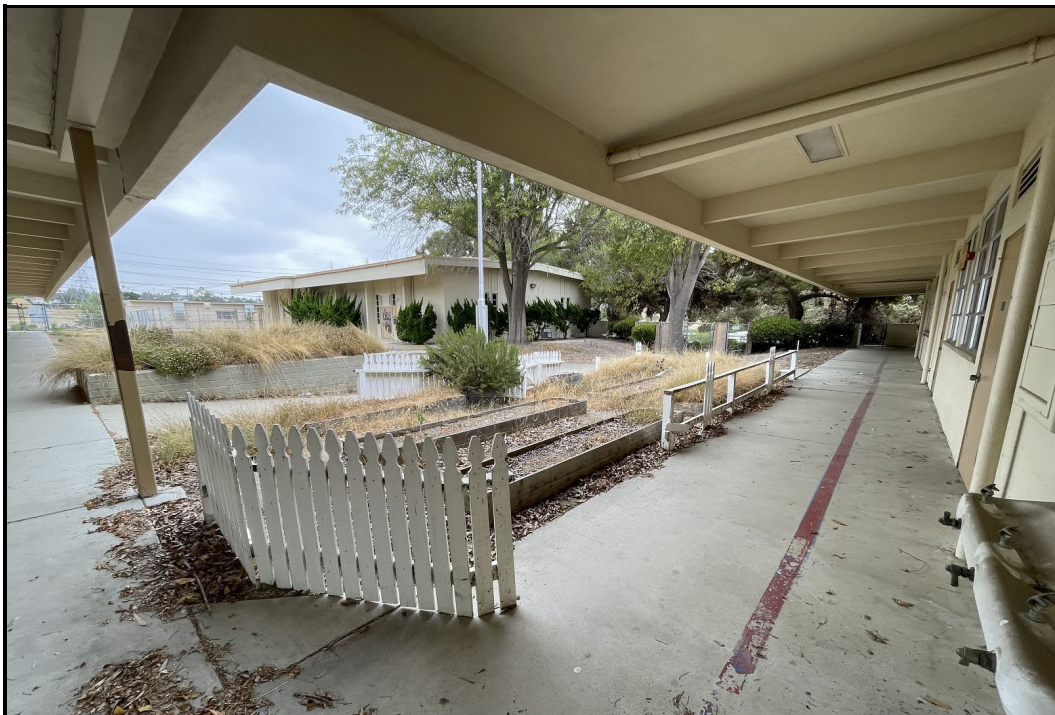
PHOTOGRAPH 8 Overview of School Office Building and Typical Planter Areas from Breezeway within Southwest APE Portion, Looking Northeast
