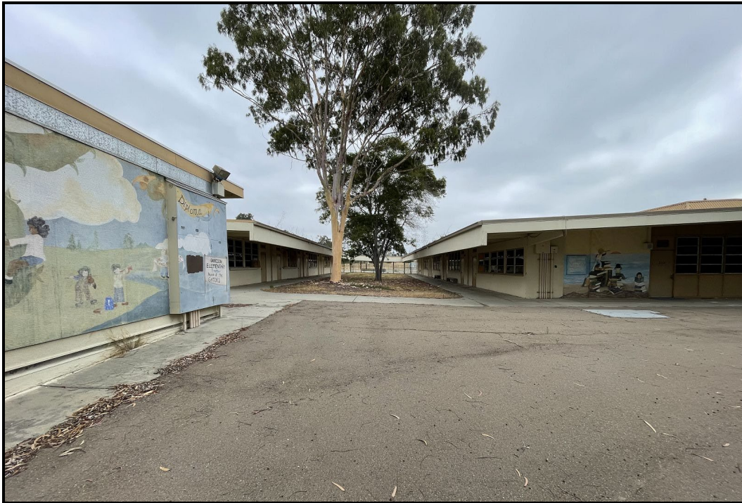
PHOTOGRAPH 7 Overview of Typical Educational Buildings, Breezeways, and Hardscape within the Southwest APE Portion, Looking Northeast
