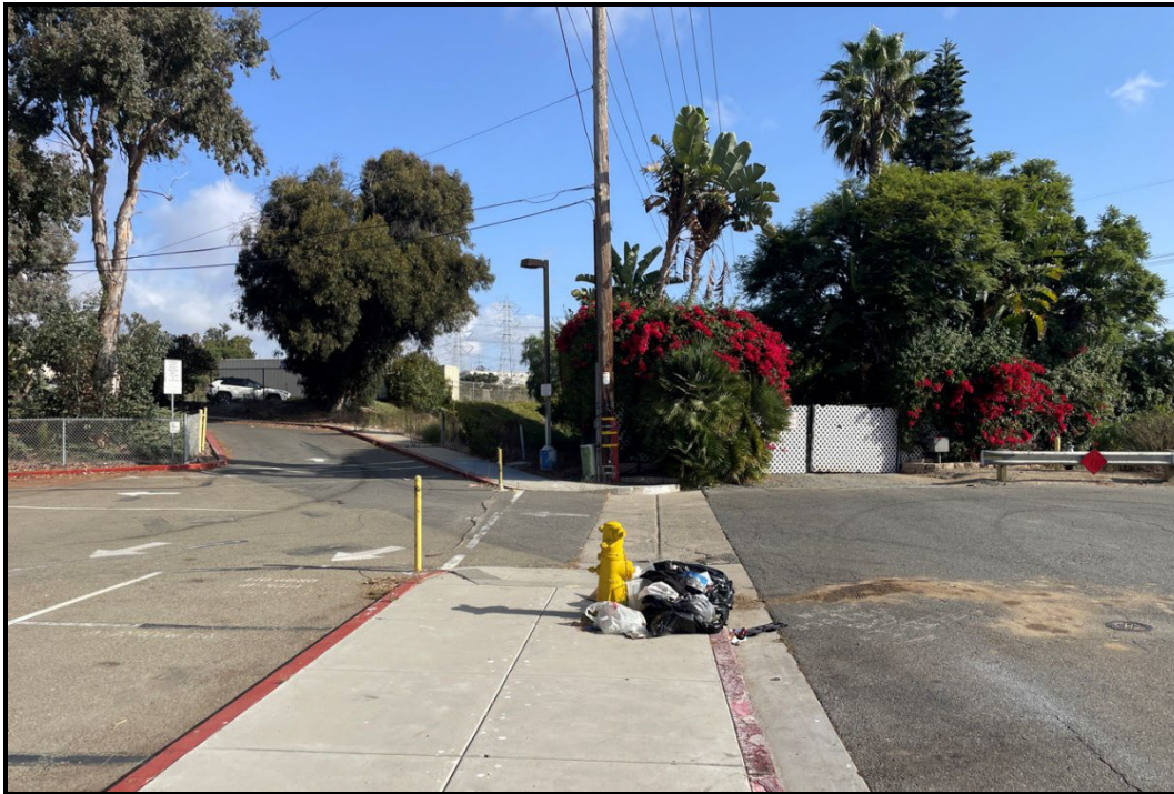
PHOTOGRAPH 5 Overview of Southern End of Off-Site Access Road Grading Area, Looking Northeast
