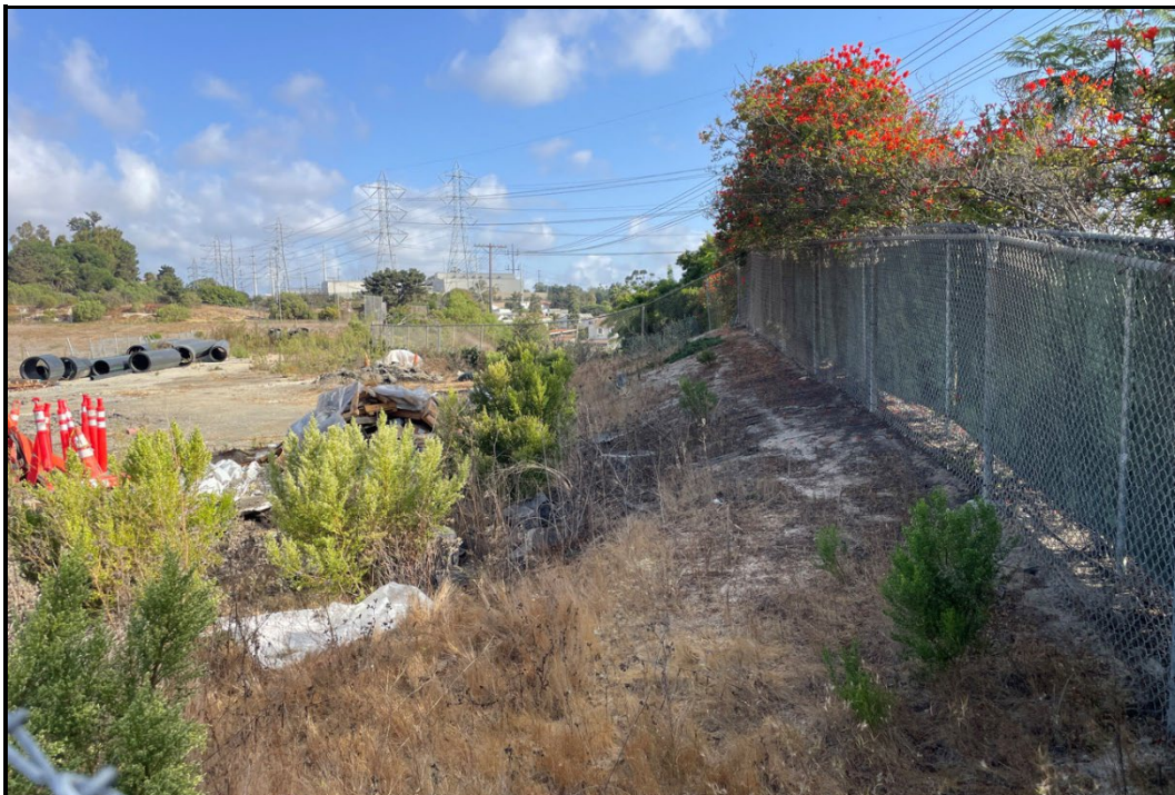
PHOTOGRAPH 6 Overview of Eastern APE Boundary within Off-Site Access Road Grading Area, Looking Northeast
