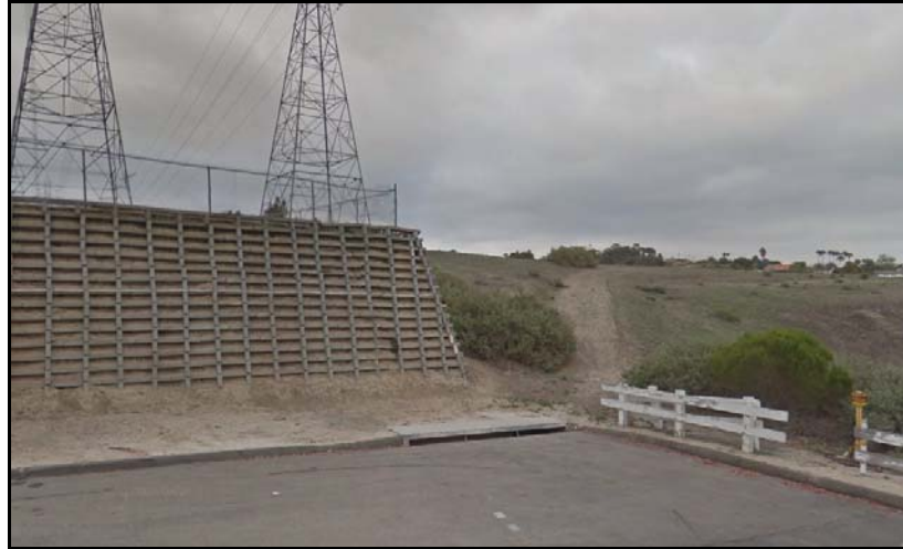
Figure 8: Existing curb inlet at terminus of Via Las Rosas (Outlet 2). Photo: Google Map.
