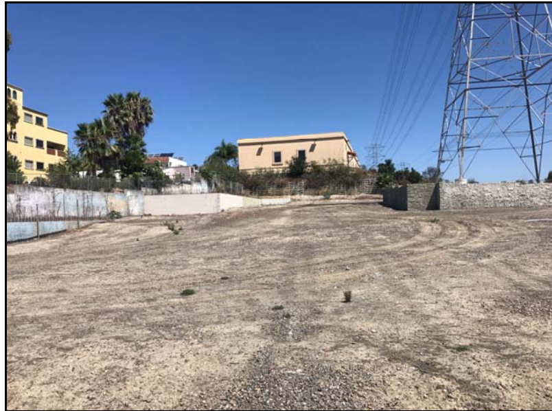
Figure 4: View of "toe" from south to north. Segmented retaining wall back left. Transmission tower to the right.
