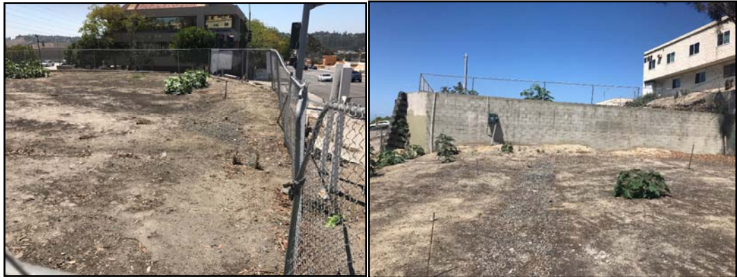
Figure 3: View from N to S of top of the "stem" graded pad adjacent to El Camino Real (left). View from driveway of retaining wall bounding graded pad above (right).
