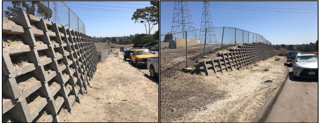
Figure 2: Existing crib walls on Via Las Rosas
