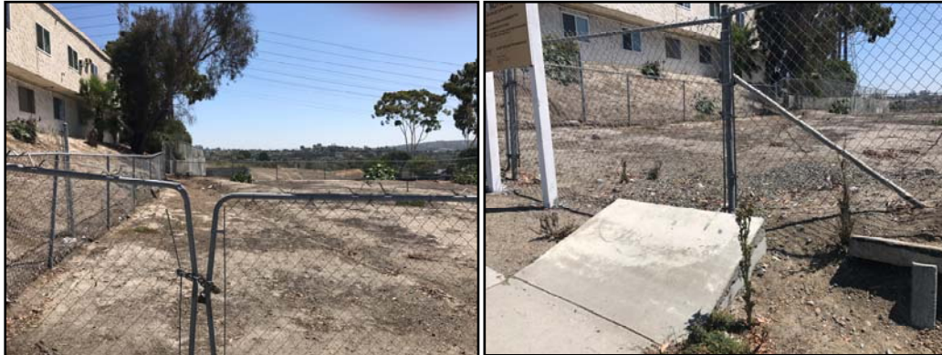
Figure 9: Natural swale (left) that conveys offsite runoff through A3 to Outlet 1 (right).
