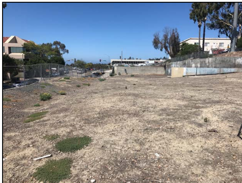
Figure 5: View of "stem" from east to west. Retaining wall in the background and to the right.
