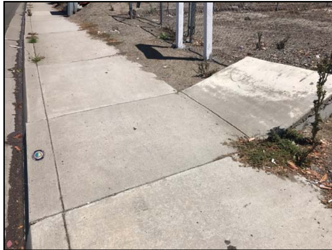
Figure 6: Sidewalk drain on El Camino Real (Outlet 1).
