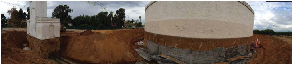
Rehabilitation of the Fire Mountain Reservoir
