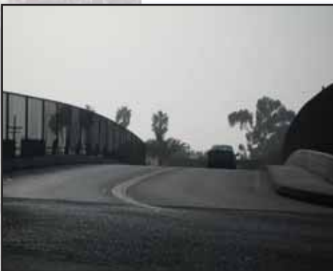
Brooks St/Division Street Bridge at I-5
