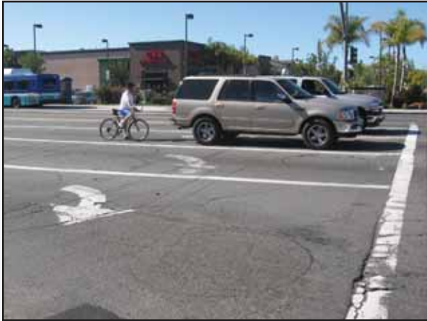
Two right-turn only lanes with no bike lanes at the intersection (Douglas Drive at North River Road)
