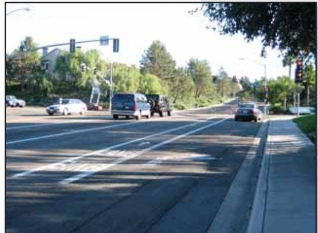
A correctly installed bike lane (Lake Boulevard at Cannon Road)
