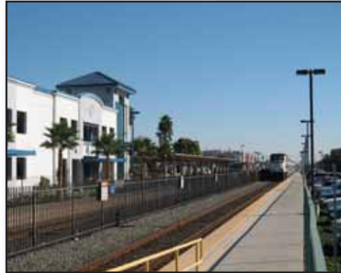
Oceanside Transit Center
