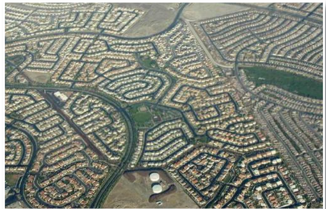
3C) A variety of barriers exist in the curvilinear and hierarchical street patterns of many suburbs. These should be avoided since fixing them later is very difficult. Photo credit: Michael Ronkin
