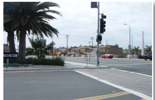
Higher contrast crosswalk materials and striping can be seen from a distance
