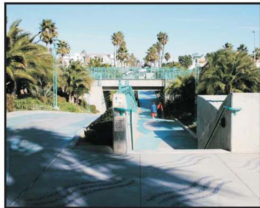
Pedestrian undercrossing at Pierview Way
