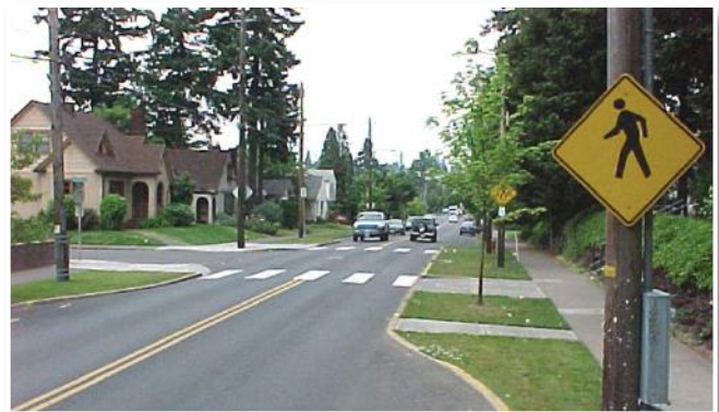
14S) This crossing is on a one lane in each direction street with curb extensions, striping, signage and trees that all help to slow a driver down. There is no multi-lane, multi-direction threat to this use of an uncontrolled mid-block crossing. Photo credit: Portland Office of Transportation
