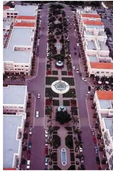
5C) Mixed use compact development supports both transit and walking by providing destinations within short distances of trip origins. Photo credit: Dan Burden
