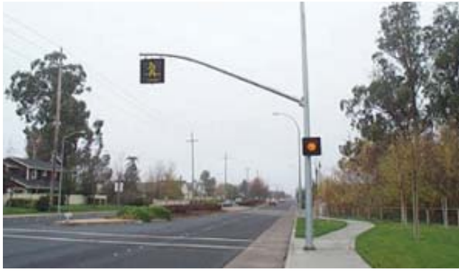
11S) This signal uses both a pedestrian crossing symbol as well as a red light when actuated. Photo credit: Michael Ronkin
