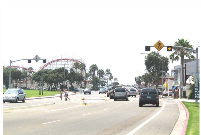
10S) A number of flashing pedestrian crossing warning signs are used throughout the region. Other solutions may be more appropriate where multi-lanes of travel on high volume streets exist. This crossing has visible signage and crosswalks along with a median refuge. Improved street lighting and advance stop bars could increase safety, but a pedestrian actuated traffic signal would provide for the safest condition. Photo credit: Mike Singleton
