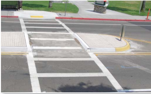
1S) A good example of a median refuge that provides access without ramps and protects a walker unable to make it across. Photo credit: Andy Hamilton
