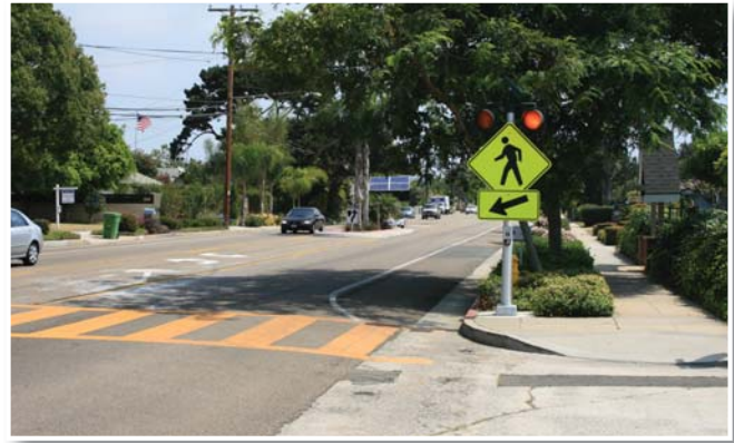
14S) If traffic control is not provided at an intersection, signage and striping along with a center pedestrian zone marker may help to make these crossings as safe as possible. This type of sign may require changes to existing policies, though it is allowed under MUTCD. Photo credit: Joe Punsalan
