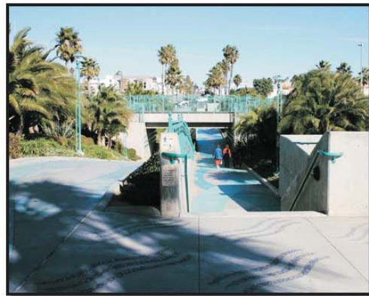
Pedestrian undercrossing at Pierview Way
