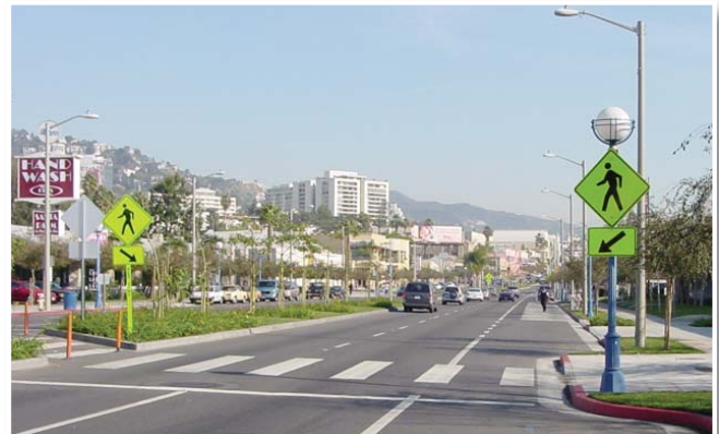
5S) Adequate lighting, pop-outs, the latest MUTCD approved signs and high visibility markings are essential for non-controlled multi-lane mid-block crossings. Note the stop bar should be located at least 15 feet from the actual crosswalk (see image on right). Photo credit: Michael Ronkin
