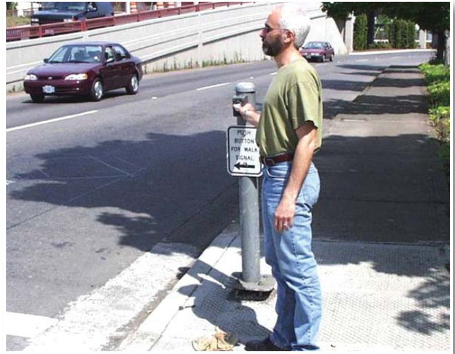
2A) Pole mounted pedestrian signal actuator placed in accessible area next to the curb ramp. Photo credit: Michael Ronkin
