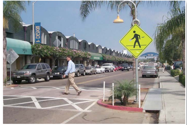
4S) Raised crosswalks (speed tables) provide clear signs of a pedestrian crossing but need to be limited to lower speed, lower volume streets. Photo credit: Andy Hamilton
