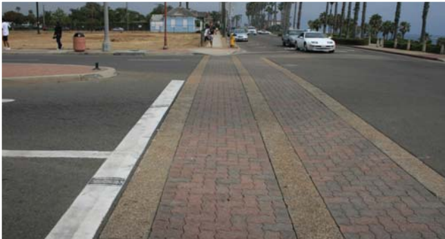
3S) Increased visibility can be obtained through a change of paving materials and striping. Photo credit: Mike Singleton
