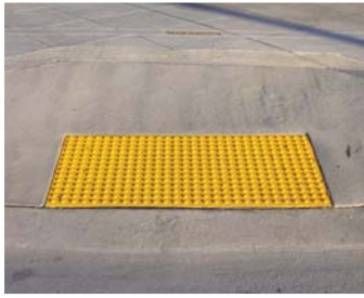
1A) Typical Two Directional Curb Ramp (note: tactile strips and truncated domes needed but not shown). Photo credit: ITE Pedestrian Bike Council
