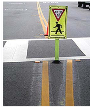
14S) This type of crossing should only be used on streets with one lane each direction or two one way lanes. The center marker is collapsible. It works to slow traffic and concentrate attention on the crosswalk. Photo credit: ITE Pedestrian and Bike Council
