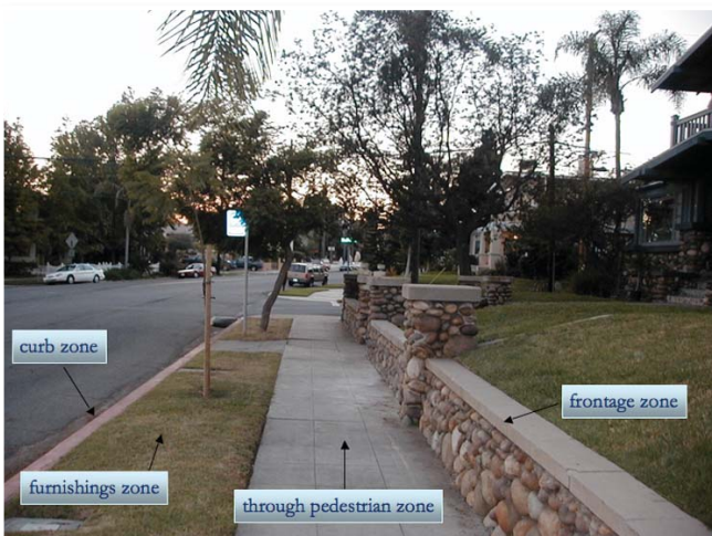
1W) Residential area widths should be at least 5' in width but no more than 10'. A walkway can feel smaller or larger depending on adjacent walls or fences and the presence of a landscape buffer. Photo credit: Andy Hamilton
