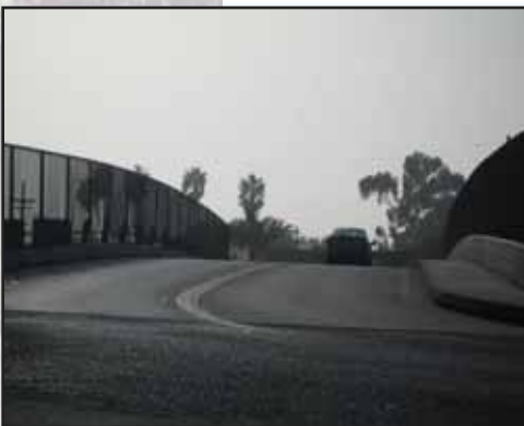
Brooks St/Division Street Bridge at I-5
