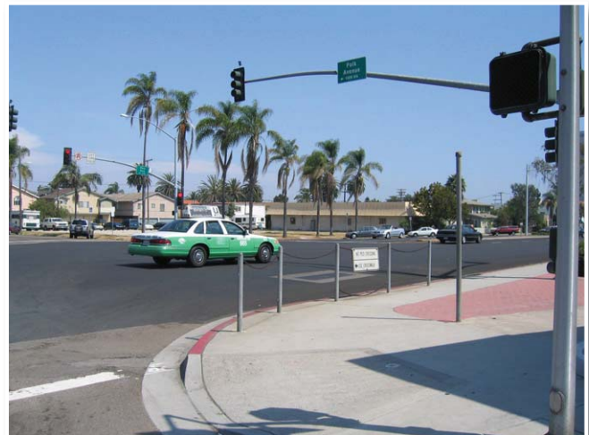
7C) There are valid reasons for closing one or more segments of an intersection including intersection geometry, such as shown above. Photo credit: Mike Singleton
