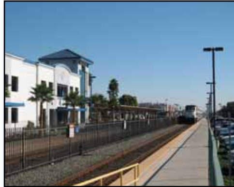
Oceanside Transit Center
