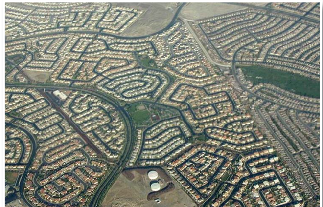
3C) A variety of barriers exist in the curvilinear and hierarchical street patterns of many suburbs. These should be avoided since fixing them later is very difficult. Photo credit: Michael Ronkin
