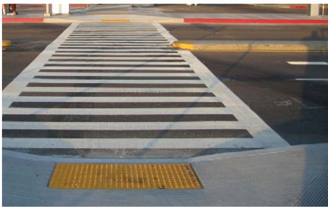
3S) Certain urban areas (that are pedestrian dominant) should utilize high visibility markings in the entire intersection. Photo credit: Michael Singleton
