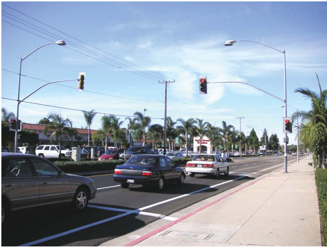
13S) This mid-block crossing utilizes standard traffic signals, a stop bar, ladder style crosswalks, median refuge and a pedestrian controlled actuator. Photo credit: Mike Singleton
