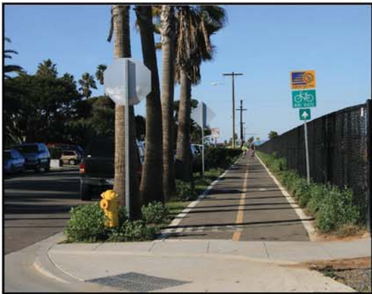
Multi-use path along Myers Street
