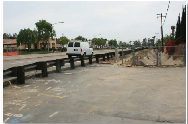
16S) As a last resort, barriers may be required to protect pedestrians along high speed streets, especially on high speed horizontal curves. Photo credit: Mike Singleton
