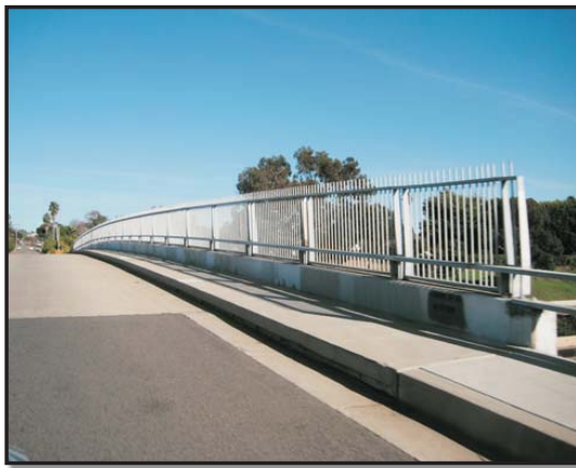
Street with sidewalk connection over Interstate 5
