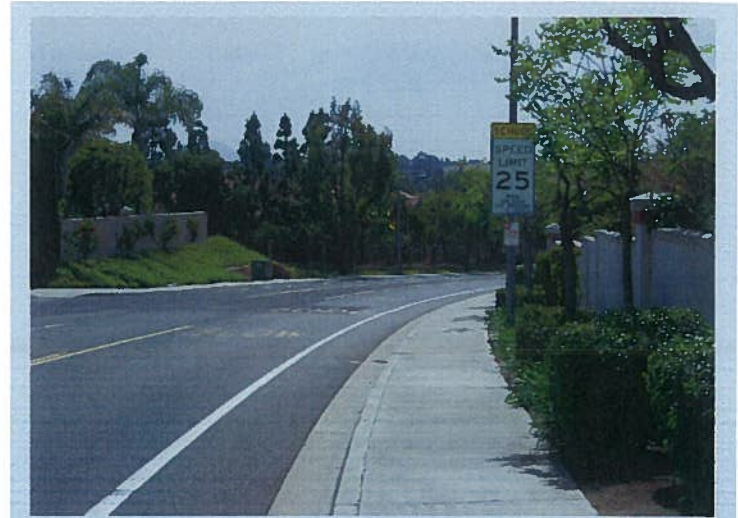
Via Rancho Road, Oceanside
