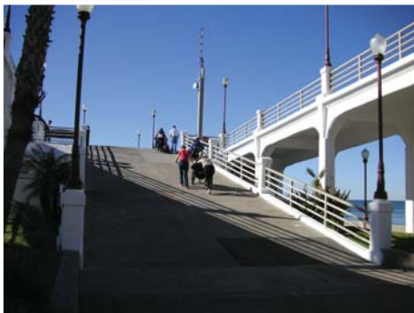
Older segments of the Oceanside Pier present challenges to disabled visitors
