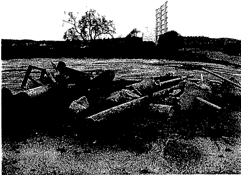
3. North view near southwest portion of property with pile of concrete and metal foundations.
