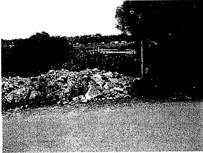
1. West view near southwest portion of property with pile of concrete.
