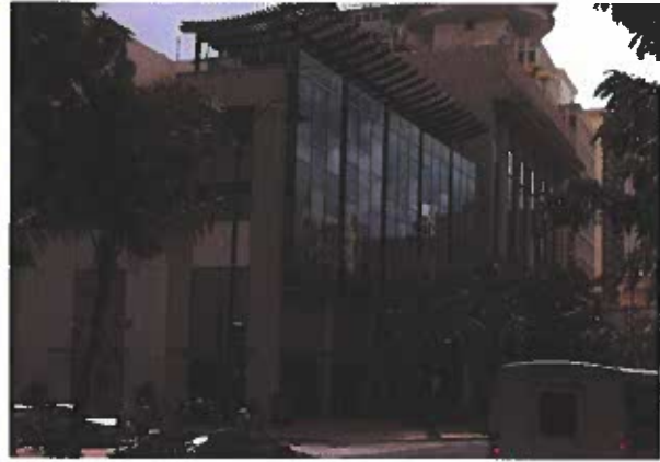
Example of Public Parking Structure
