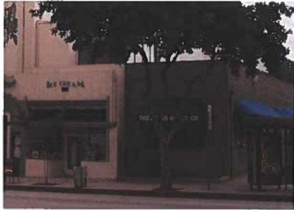
Example of Main Street Retail/Office
