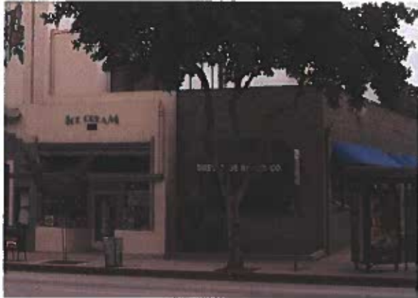
Example of Main Street Retail/Office
