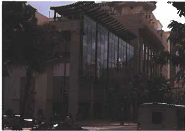
Example of Public Parking Structure
