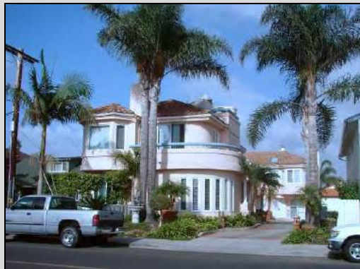
Figure II-3.5e: Use upper-story setbacks or partial indentations for upper-story features, such as balconies, outdoor moldings or cornices, to accentuate the horizontal levels of a building.
