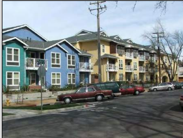
Figure II-2.3b: Don't do this - Design a tall sidewall to be placed near a property line when it will be adjacent to similar walls on the neighboring site.
