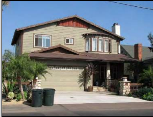
Figure II-3.5c: Use a few simple, well-proportioned masses accented with a few smaller elements, such as bay windows or dormers.
